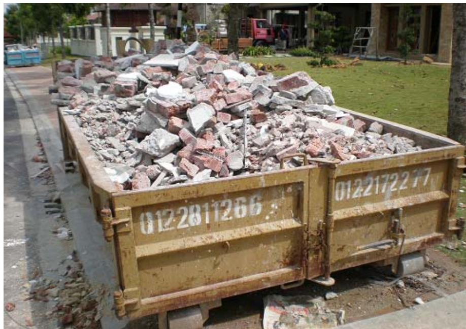
Figure 5.4: Brick that can be reuse as hardcore material
