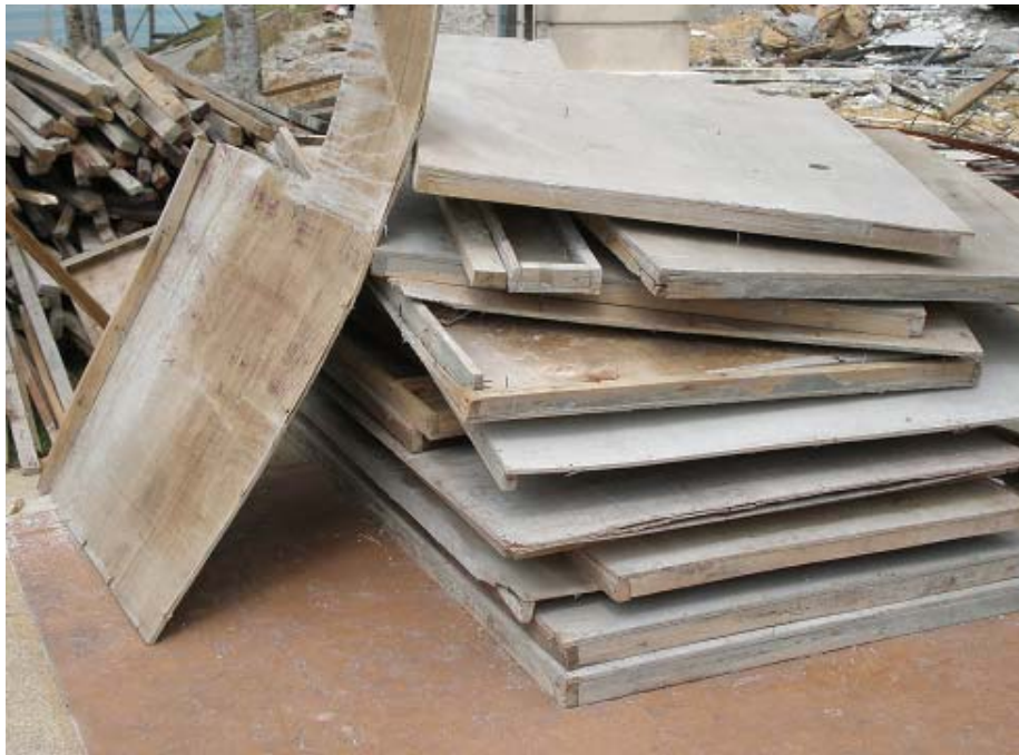
Figure 5.1: Formwork major contribution in construction waste
